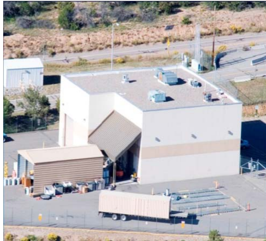
RANT Facility, TA-54
