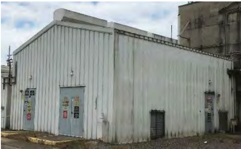
235-1F Refrigeration Building
