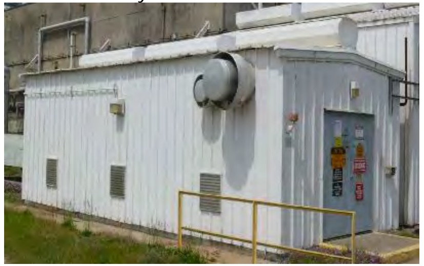
235-2F Refrigeration Building
