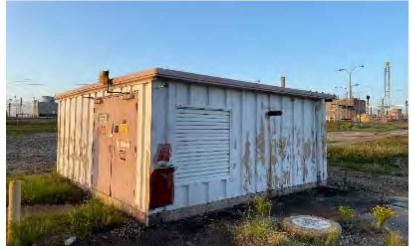
607-3F Sanitary Lift Station
