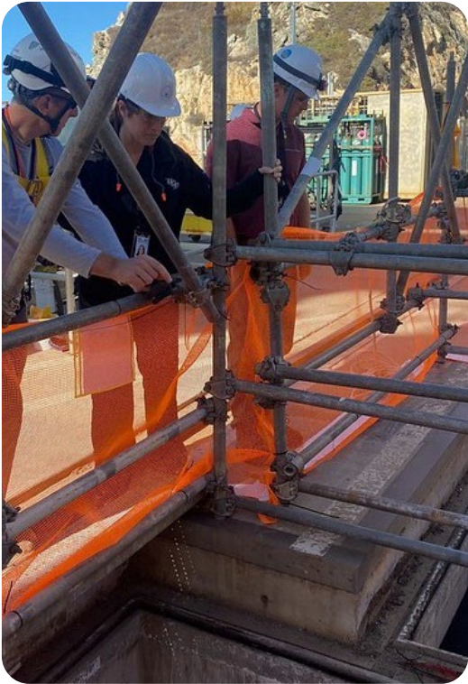
NRC renewal inspection of Diablo Canyon plant's electrical cable box
