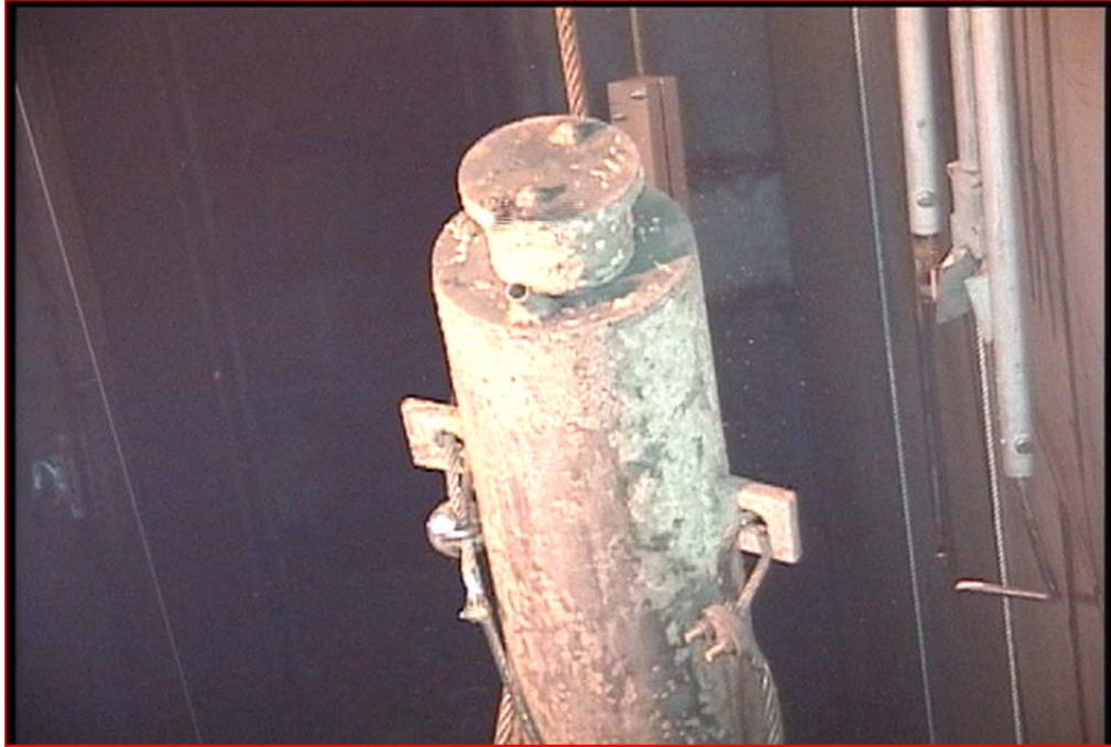
Figure 13. Failed element container with evidence of pitting.
