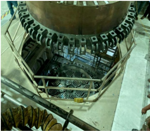
Opening the process gas filter on the Integrated Waste Treatment Unit at INL. (Source: 33 rd Annual Report to Congress)
