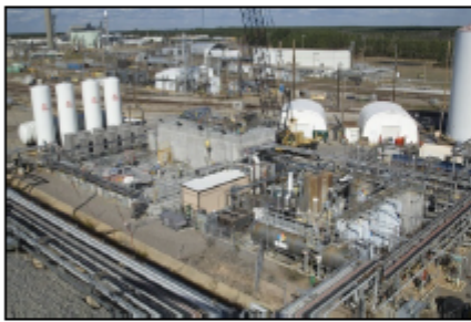
Savannah River Site, Salt Waste Processing Facility, (Source: srs.gov)
