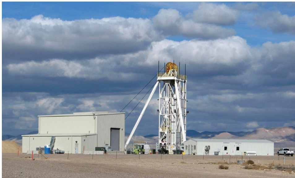
U1h Hoist at the Nevada National Security Site U1a Complex
