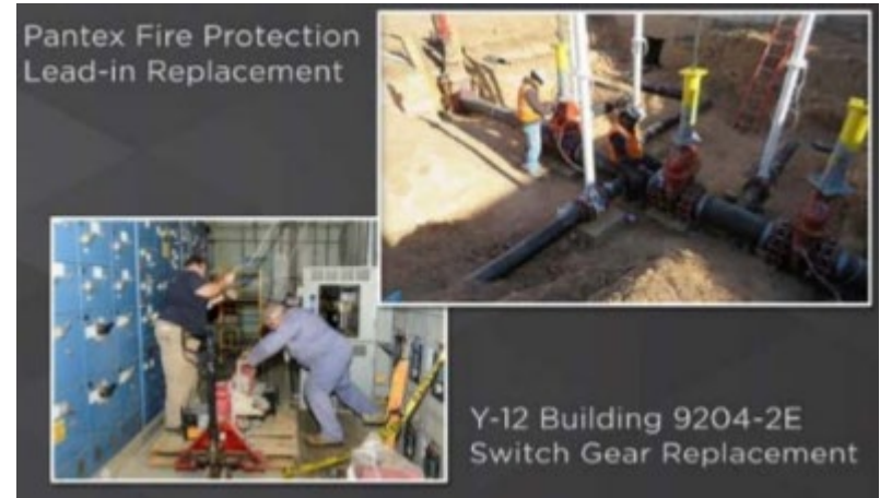
Y-12 and Pantex Infrastructure Upgrades
