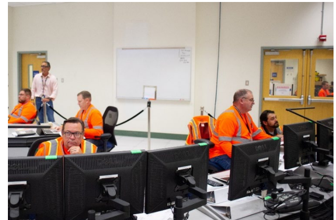
LAW Facility Control Room
