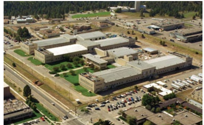
Los Alamos Chemistry, Metallurgy, and Research (CMR) Facility
