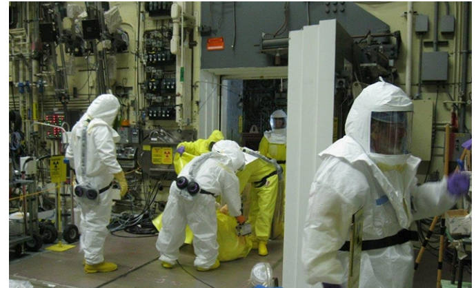
Workers bag waste out of the Building 324 Hot Cell Airlock
