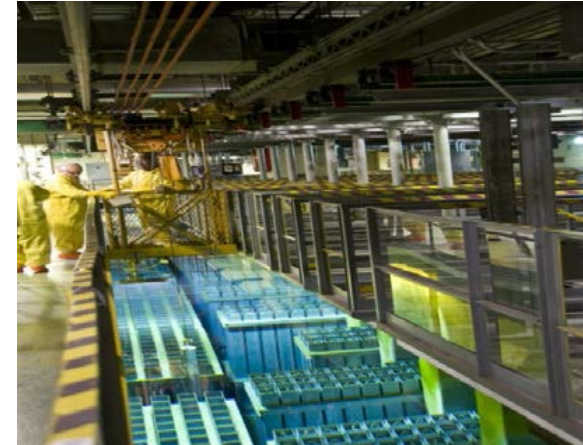
Savannah River Site (SRS) L-Area Spent Fuel Basin
