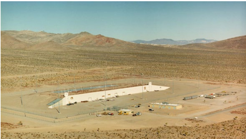
Device Assembly Facility Structure
