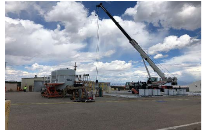
Los Alamos Area G Mobile Loading Activities
