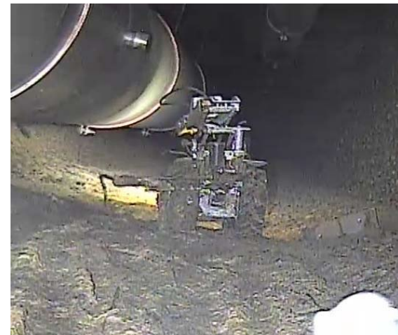
Crawler Inspection of SRS H-Canyon Exhaust Tunnel
