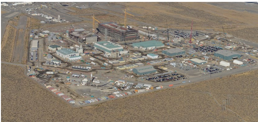
Hanford Waste Treatment and Immobilization Plant
