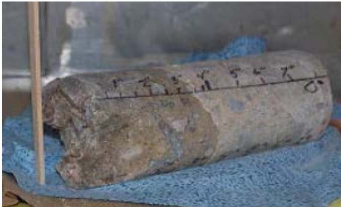
Figure A-3. Concrete core exposed to the HCAEX environment (left side of core) removed from north wall of the Personnel Tunnel.
