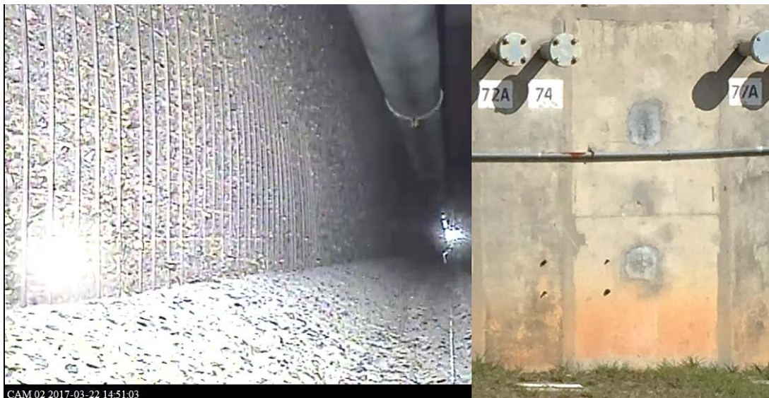
Figure A-2. Comparison of a still from the 2017 crawler inspection video of inside HCAEX Tunnel (left), and a set of two coring locations on the exterior wall of the H-Canyon Facility (right).
