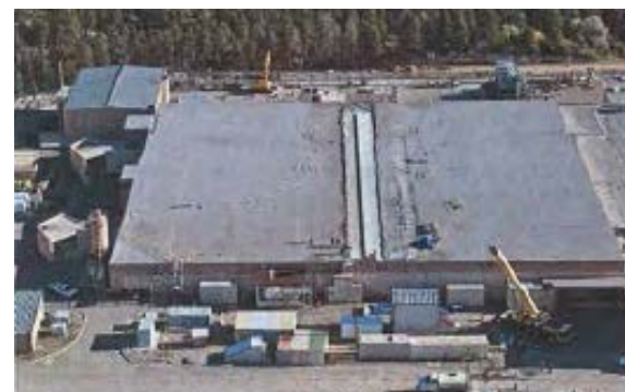
Plutonium Facility Structural Seismic Improvements
