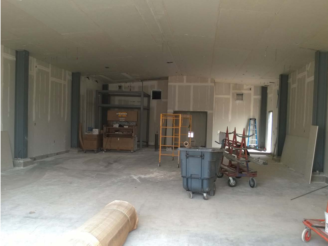
Figure C-3. Interior of typical Waste Storage Building, nearing completion of construction
