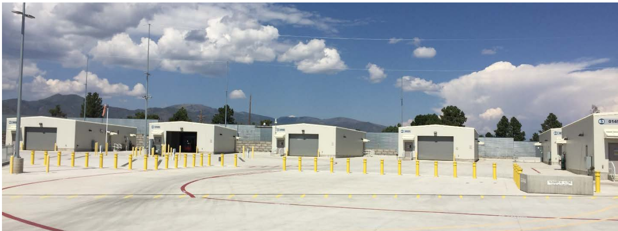
Figure 1 – Completed Transuranic Waste Facility
