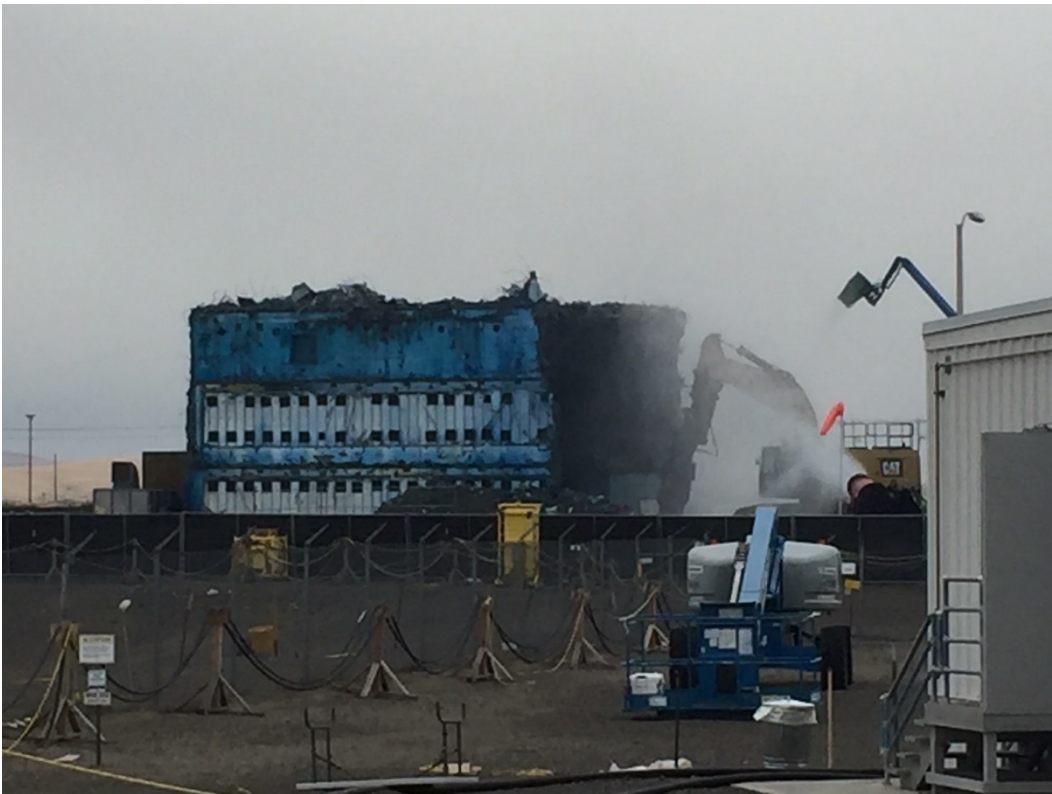
Demolition of the Hanford Plutonium Finishing Plant
