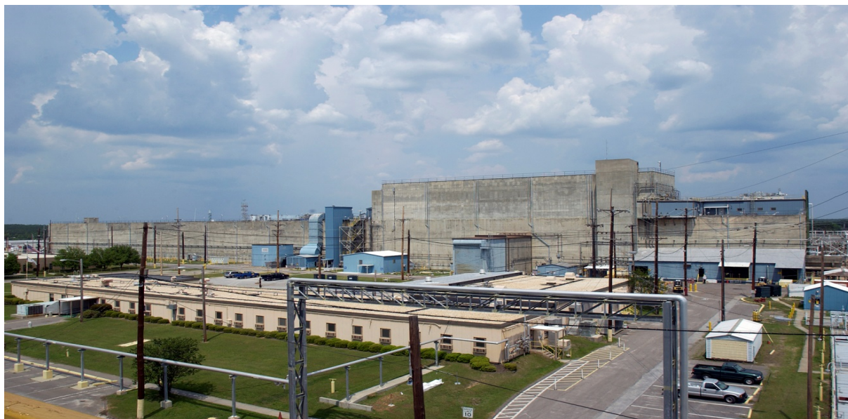
Savannah River Site H-Canyon and HB-Line
