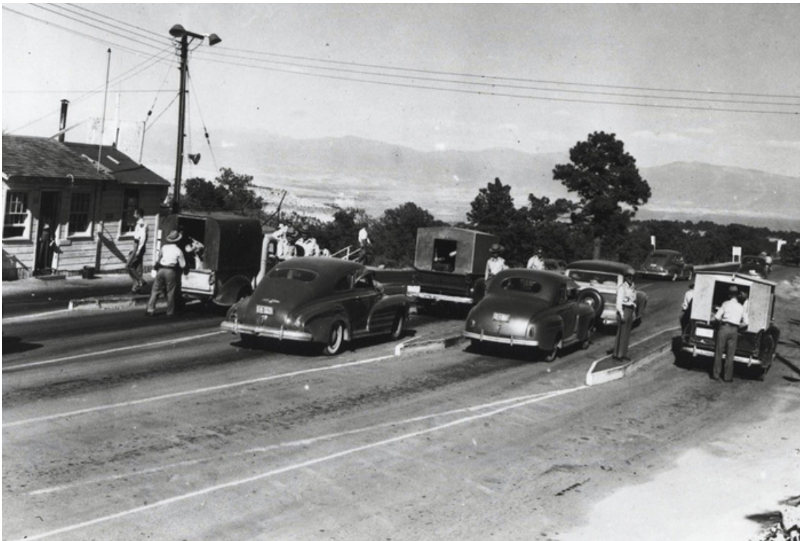
Los Alamos Main Gate, Manhattan Project
