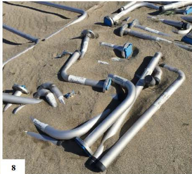
Figures A-7 to A-8. Staff review team photographs illustrating deficient storage conditions at the MHF Laydown Yard. Figure A-7 shows water accumulated inside a vessel. Figure A-8 shows additional pipe modules buried in the sand.
