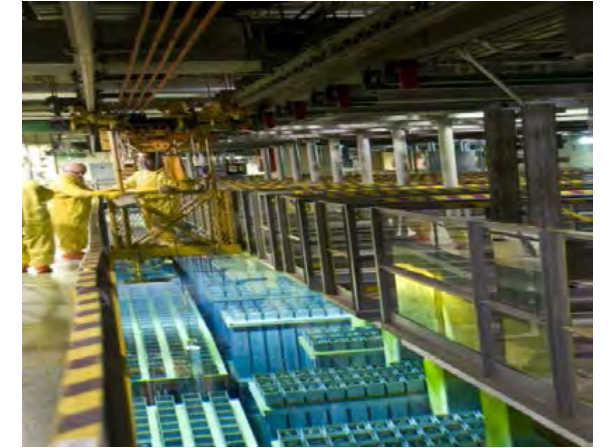
L-Area Spent Fuel Basin
