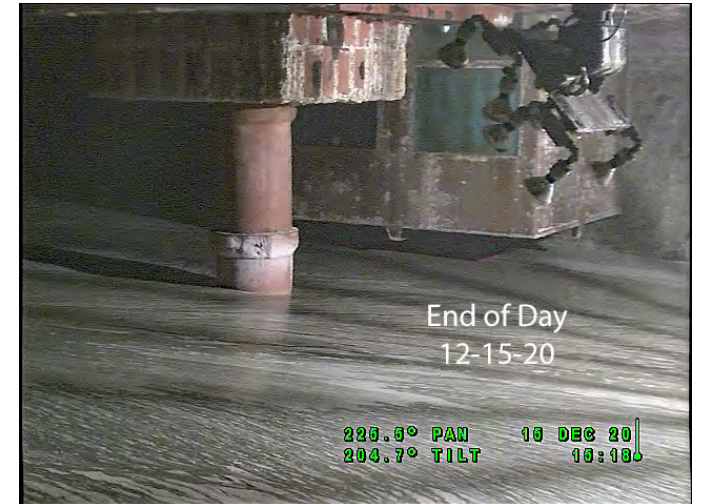
Inside 219-Z-9 Crib – December 2020
