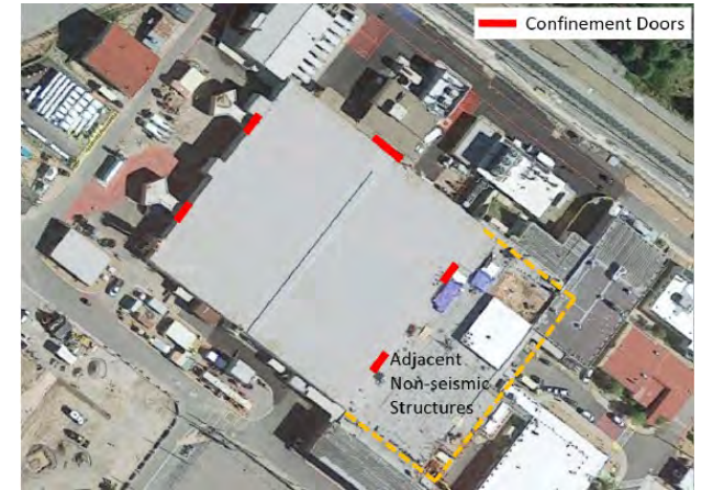
Doors in Passive Confinement for Plutonium Facility at Los Alamos
