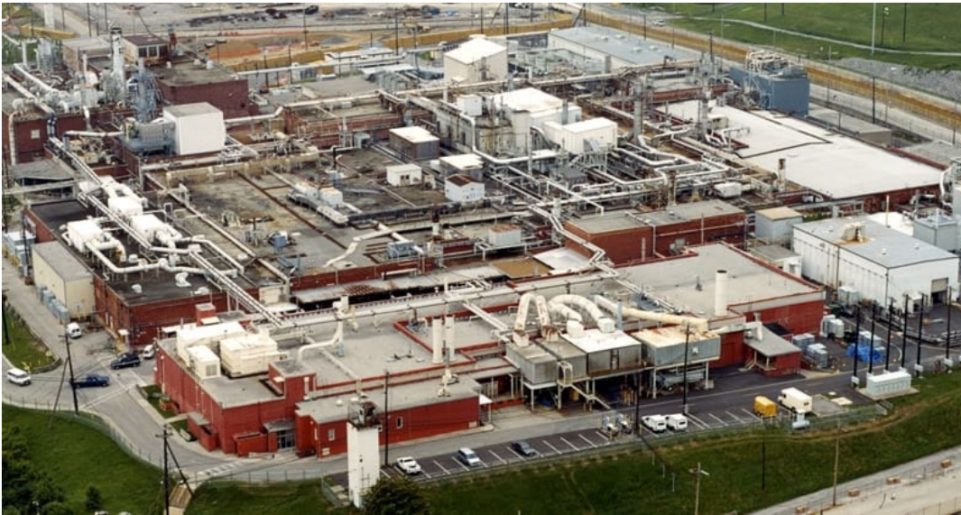
Building 9212, Y-12 National Security Complex
