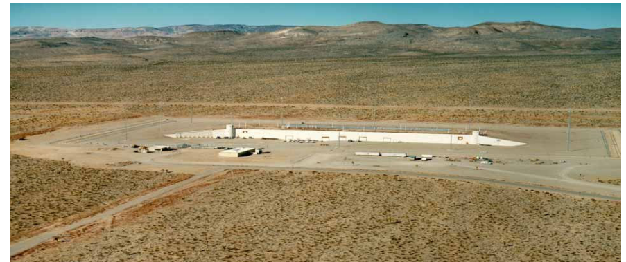
NNSS Device Assembly Facility
