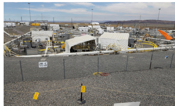
241-C Tank Farms, Hanford
