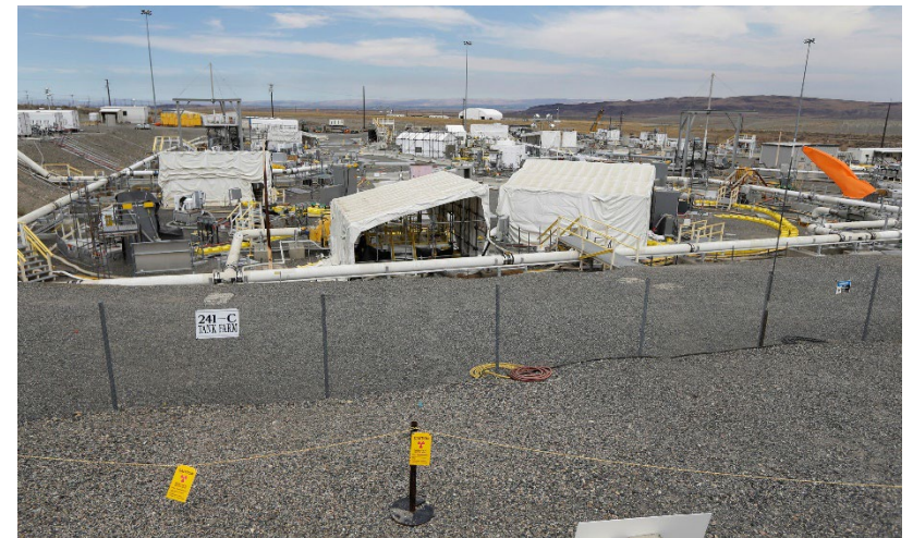
241-C Tank Farms, Hanford
