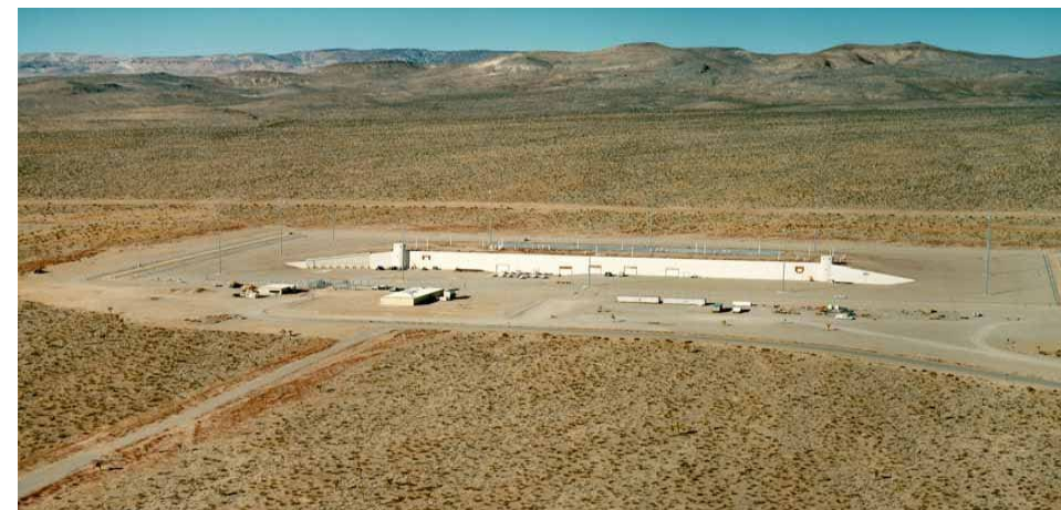
NNSS Device Assembly Facility
