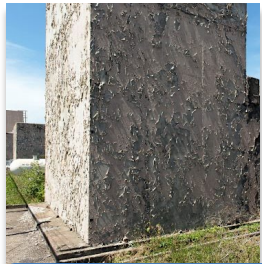
GRC Exhaust Stack Erosion FY17
